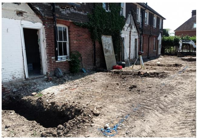
Plate 2: Foundations excavated in the eastern part of the site.
